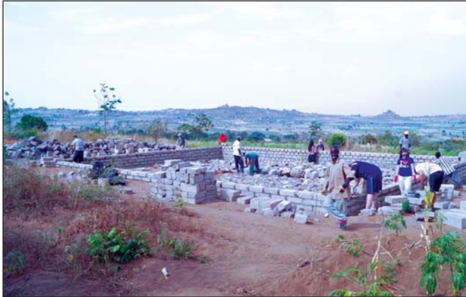
Foundations of the Doctor's house.
